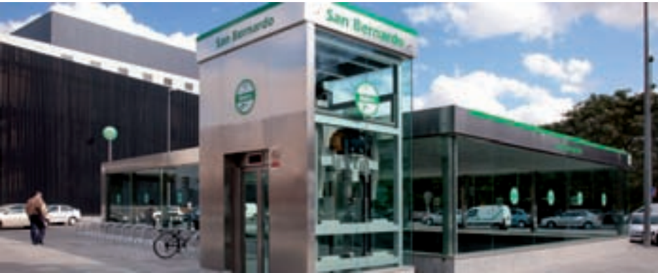
MP GLASS lift Seville metro, Seville, Spain.
